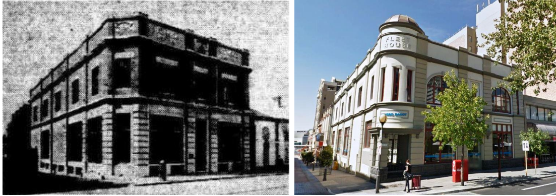
The showroom-offices Oldham designed for H.V. McKay Pty Ltd on the north-east corner of Murray & King Streets, Perth in 1924 have been highly modified. Oldham also designed a large factory for the company at Crawford Road, Maylands in 1926. ( The West Australian , 28 March 1925 p.14, Google 2014).
