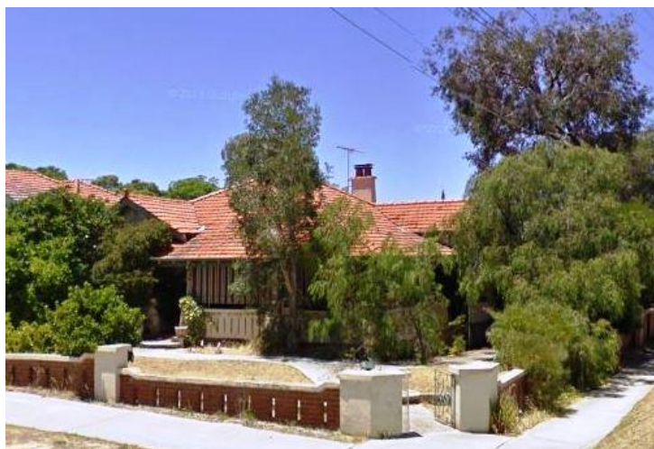
Residence designed in 1932 at 74 Smyth Road Nedlands for Alex J. McIntyre (Google 2014).
