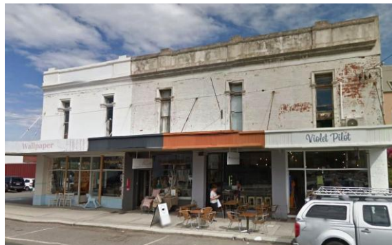
In late 1903 Ronald Oldham designed three two-storey shops & residences at Victoria Avenue, North Fremantle for Dr Kenny – they are likely to be these shops at 257-61 Queen Victoria Street - although the Kennys did own other shops in the street (Google 2014).
